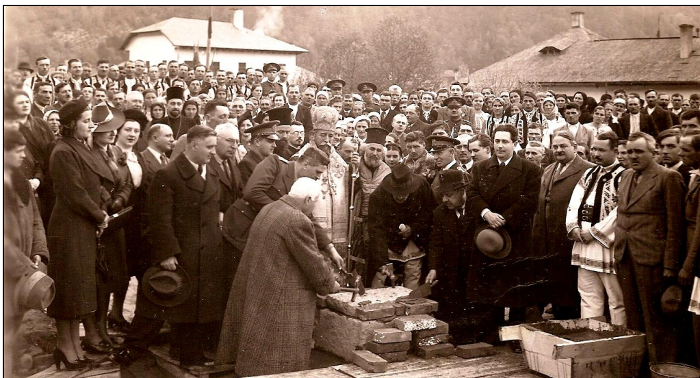
The consecration of the site and the laying of the foundation stone of the current building of the Tarcău School – 1938 (Constantin Turcan lays the foundation stone of the new school; in folk costume, Mayor T. Ailincăi)
